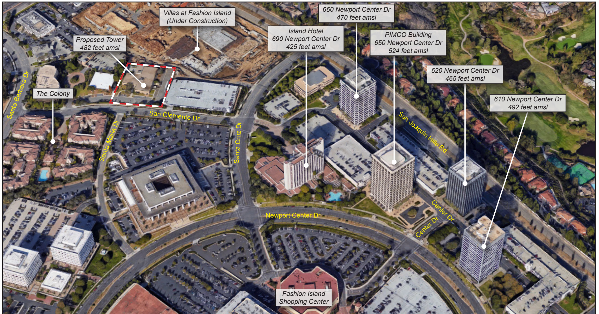
Figure 5.1-2 - High-Rise Buildings in Project Area 5. Environmental Analysis
